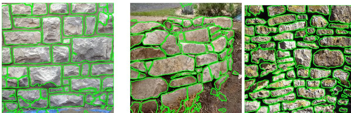
**Fig. 5.1.** Results of the proposed brick segmentation method for three difference wall images
