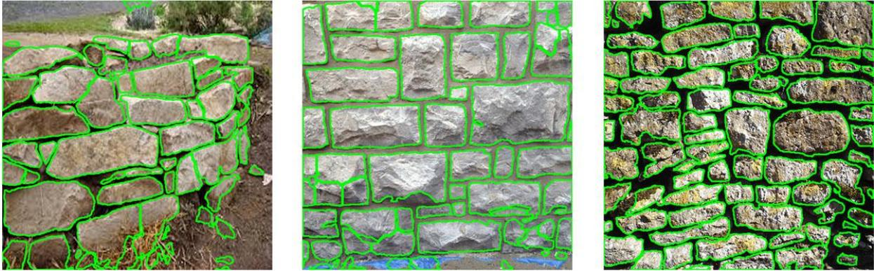
**Fig 6.** Automated brick segmentation results for different (regular and irregular) masonry wall images, using the proposed CNN and Watershed based model
